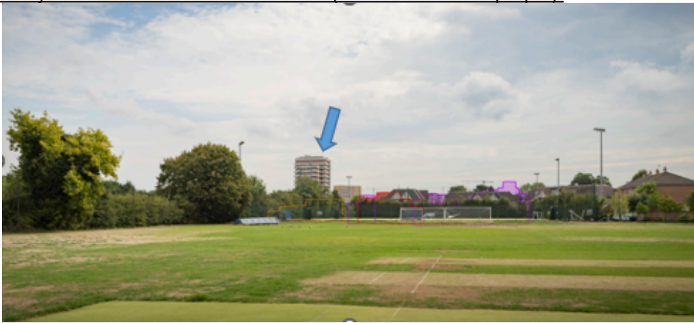
Verified wireline View 4 of block (in green) from within Ealing Common CA:
