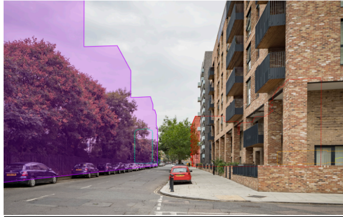
View 10 from Bollo Lane south side close to listed Acton Town Station proposed block (fully rendered) cumulatively with other consented scheme (coloured purple):
